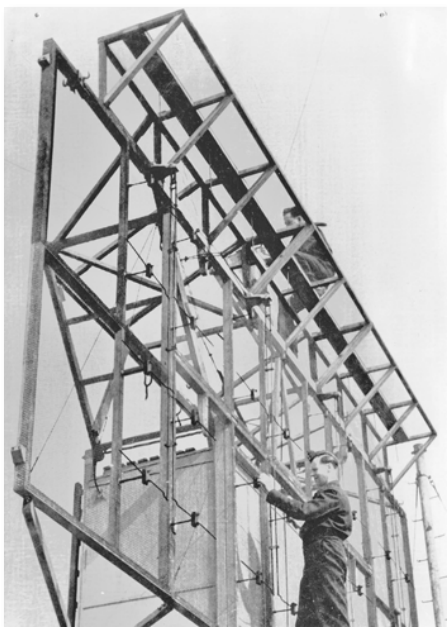
Figure 3 - Type 15 Aerial on a FDT
