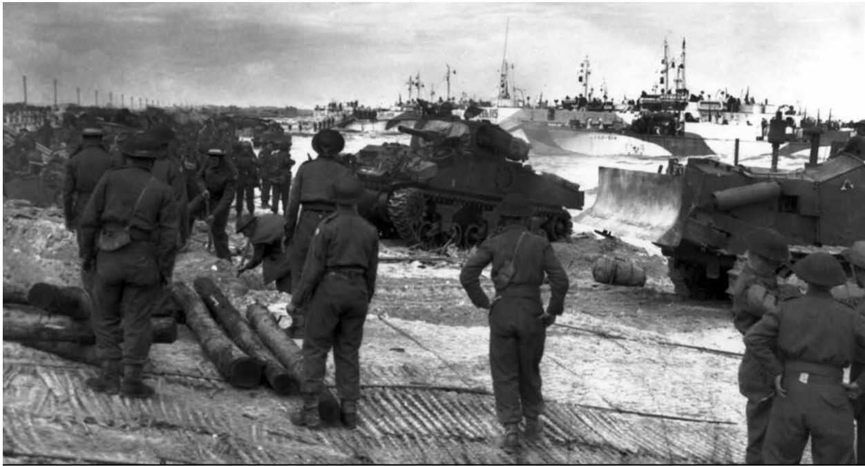
Juno Beach on the afternoon of D-Day. This is the sector at Courseulles-sur-Mer where 7th Canadian Infantry Brigade, supported by the tanks of the 1st Hussars, landed.
