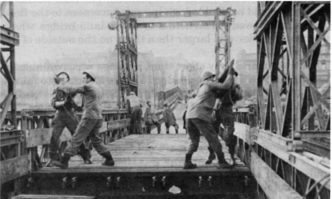
Engineers lift the bascule span of a class 70 Bailey bridge. (Engineer School Library)
